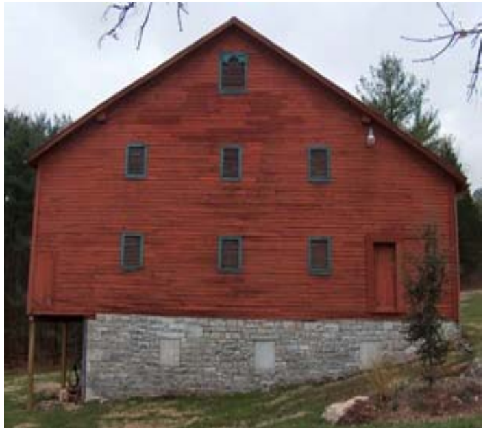
The barn sits on a slope so that the second level may be accessed easily.
