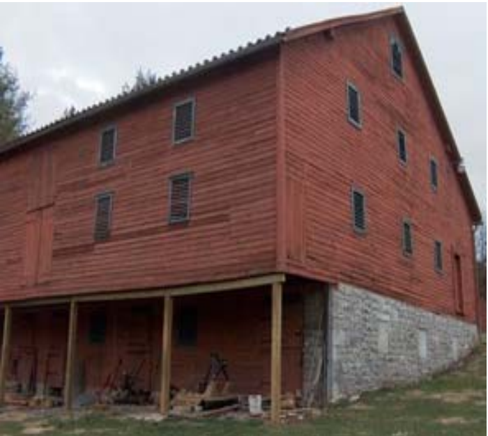
The forebay protects the livestock doors. Note the added vertical supports.
