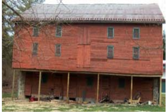
Note the levels of the barn and the eight ventilation louvers.
