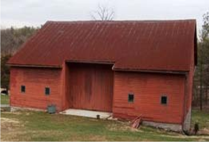
The barn is banked for easy access to upper level. This type of barn has “sheds” flanking the main doors.
